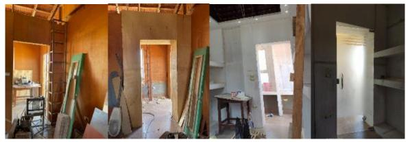
Photos n. (19) show the wall BB`before and after installing the wooden cladding, the initial paint stage, and after fixing the door.
