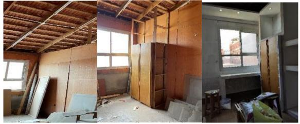
Photos n. (18) show the wall DD` and part of the wall AA`before and after fitting the storage unit, and the desk. The last photo was in the primary painting stage.
