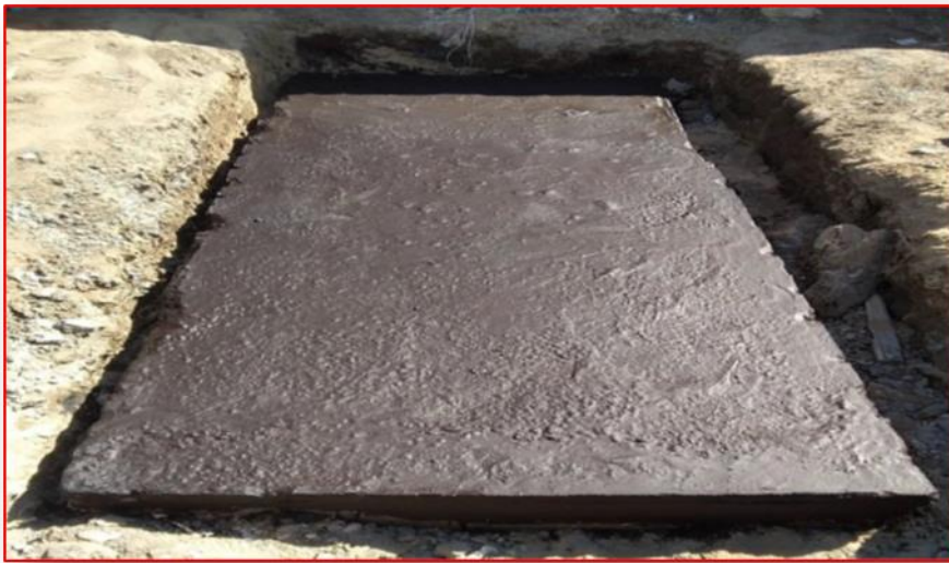
Fig (13). Shows the concrete and the dripping burlap placed on the bitumen material to protect the base from ground water
