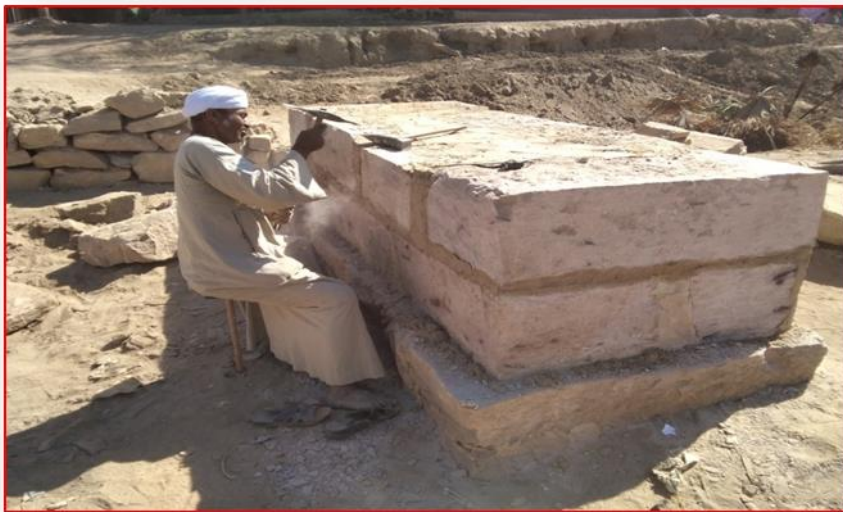
Fig (18). The shape of the first course, and the second after installation on the base and filling the gaps and joints between the stone blocks with mortar
