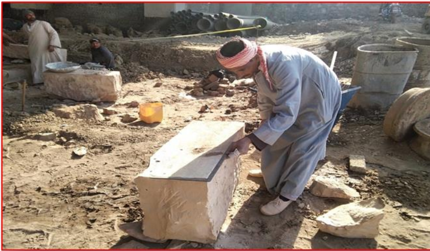
Fig (15). The work of sculptors while refining the stone blocks used in building the base (which are Nubian sandstone blocks) and determining the dimensions and sizes of each block
