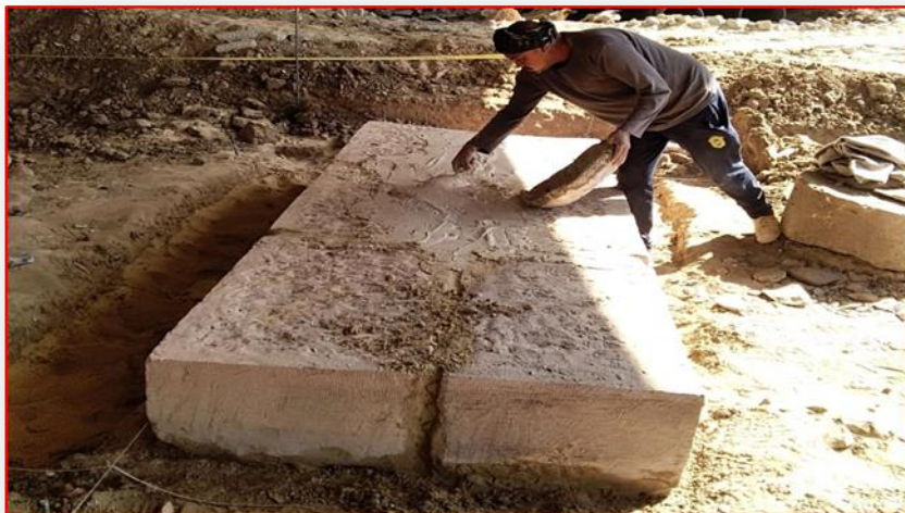
Fig (16). Placing the foundation course in the base and placing the mortar on it to connect it to the rest of the other courses
