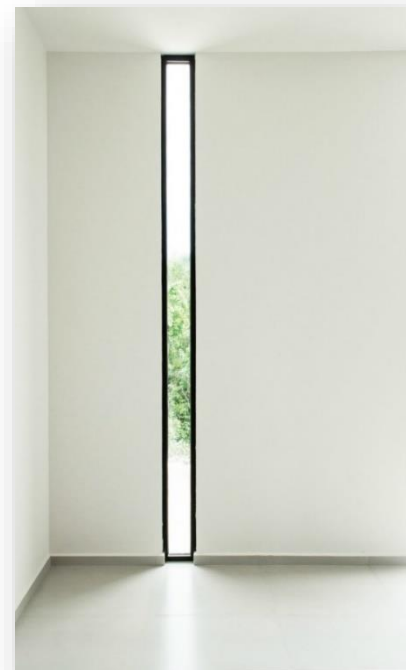
Figure (10). windows from roof to floor could provide more light especially if the room located in the south side (denfair.2017)
