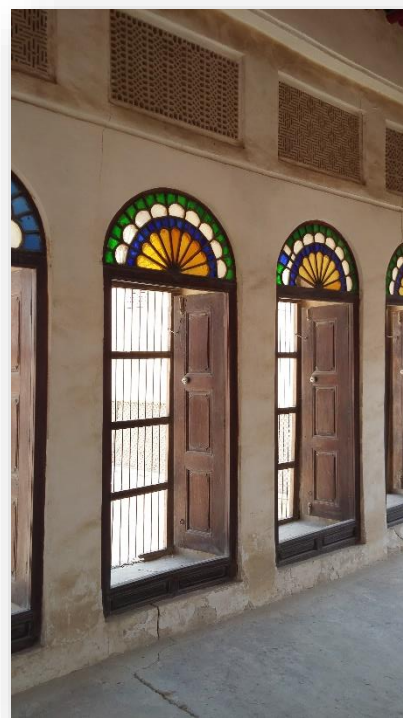
Figure (8) Traditional window of house in Muharraq, Kingdom of Bahrain - photographed by the researcher
